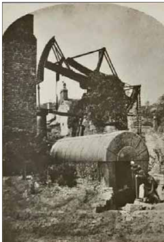
Photos by Jackson Brothers, 1861, clearly showing the boiler shaped like a covered wagon.
